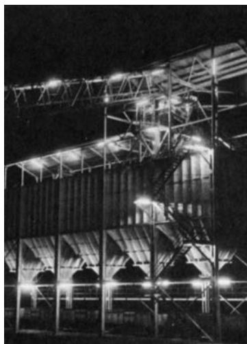
Fuel preparation plant at Mae Moh lignite mine, Thailand.
