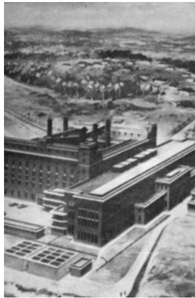
The Connaught bridge power station in Malaysia.
